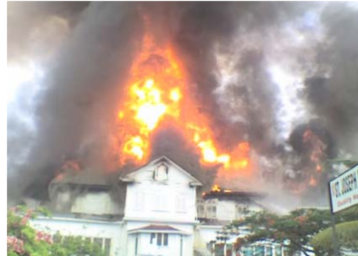
Vieux Fort, Saint Lucia, St. Judes Hospital Fire 2009
