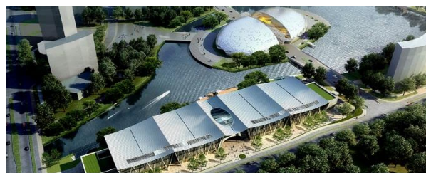
Deqing International Convention Center & Deqing International Exhibition Center
